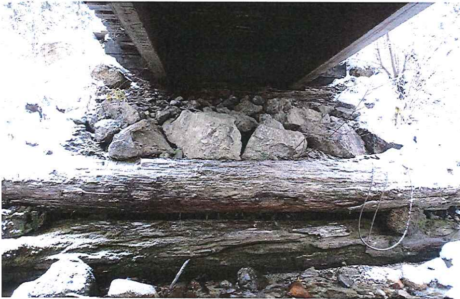
CK2015 Right Abutment
