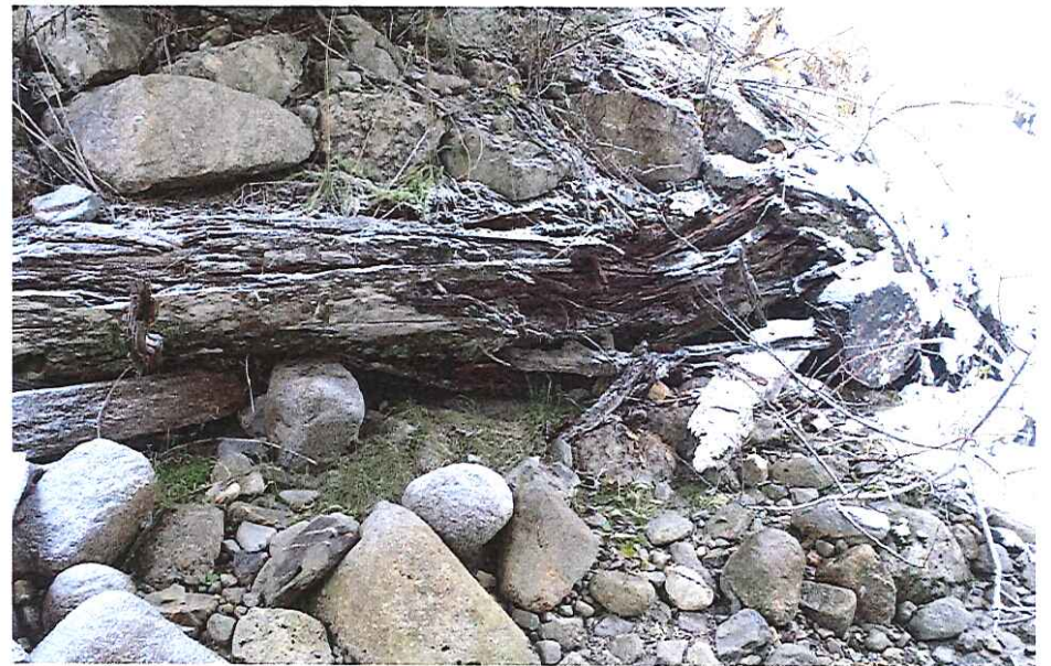
CK2015 Left Abutment crib
