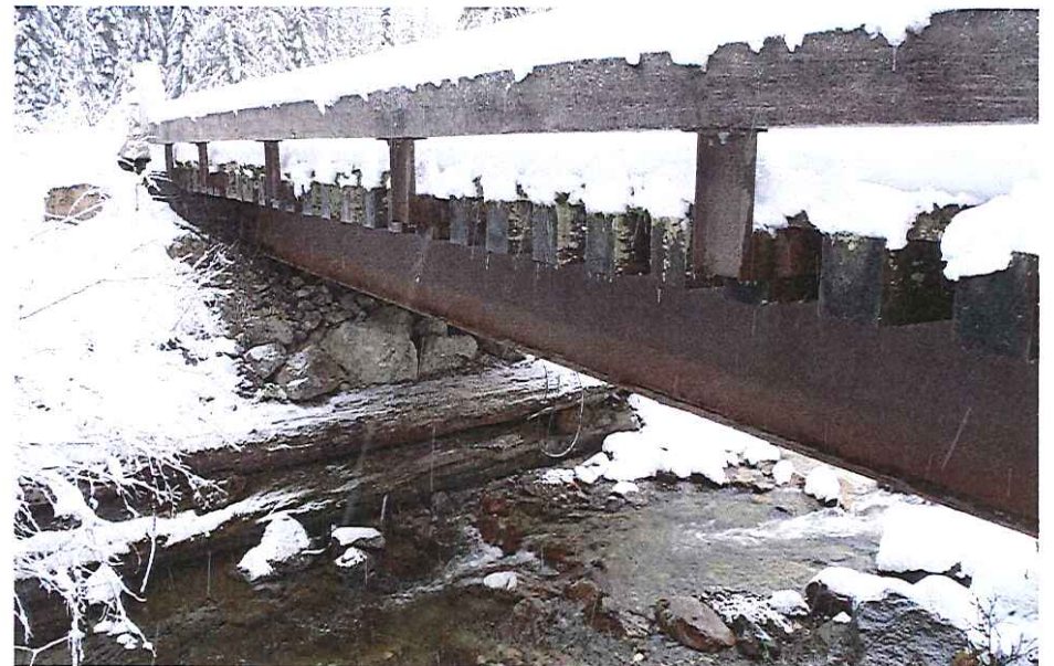
CK2015 From Downstream
