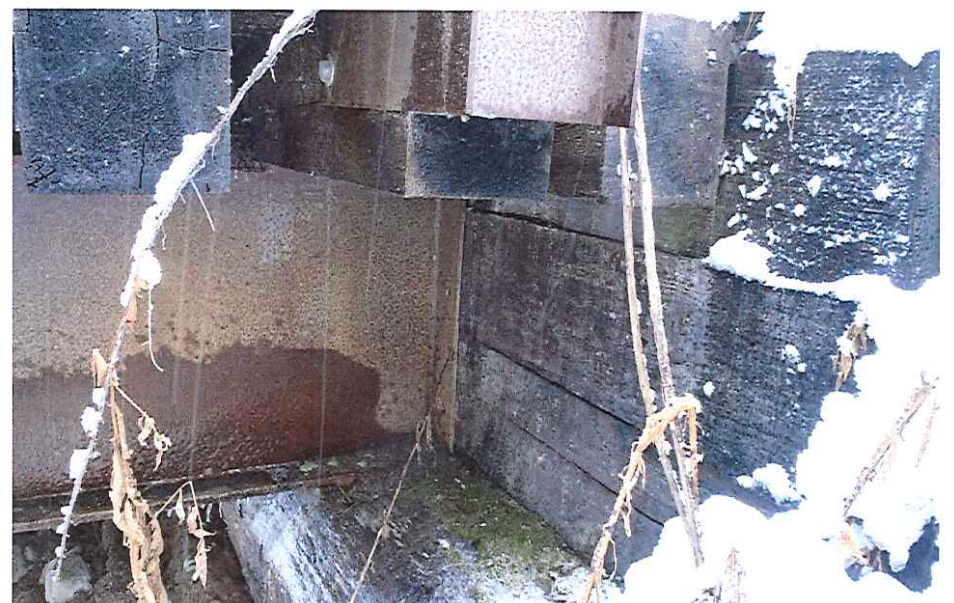
CK2015 Left Abutment Bearing
