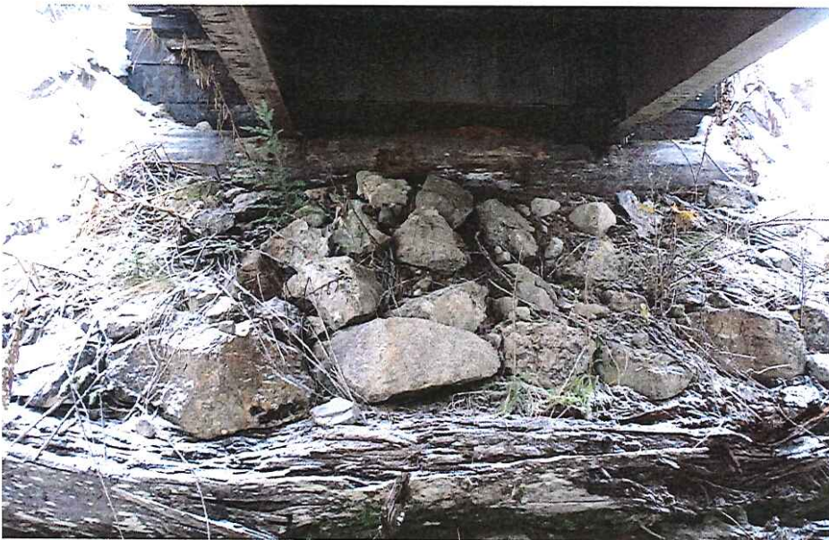
CK2015 Left Abutment
